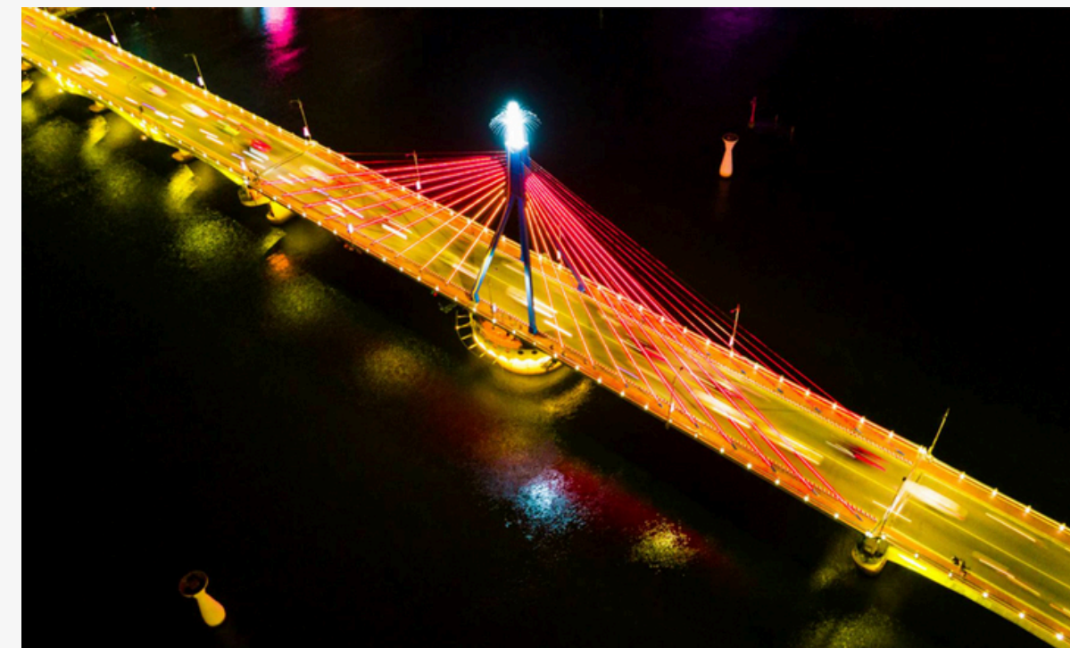
Han River Bridge Distance: ~3,2km
